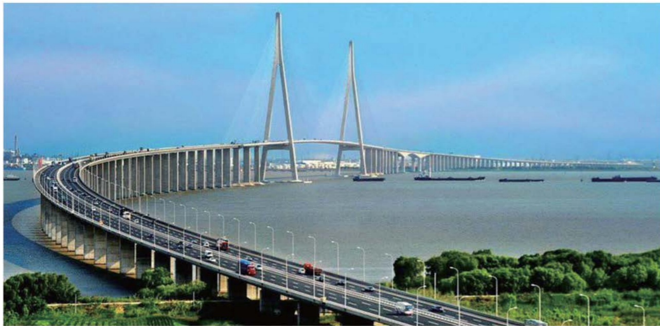
Hangzhou Bay Bridge
