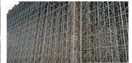
High support formwork
