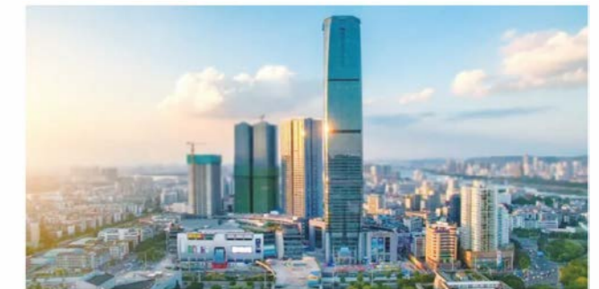
The Diwang International Fortune Center in Liuzhou, Guangxi
