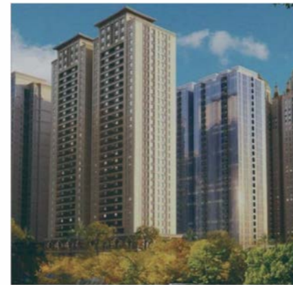
Megada Project in Indonesia
