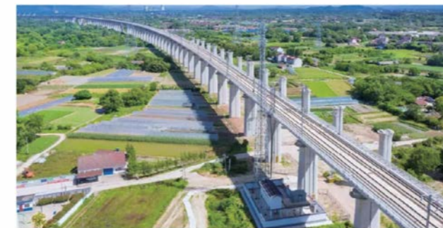
Hefei-Hangzhou High-Speed Railway Project
