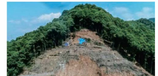
Zhejiang Jiande Slope Project
