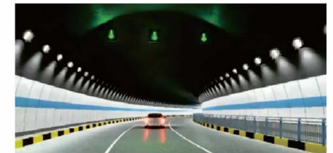
Tunnel Project in Saudi Arabia
