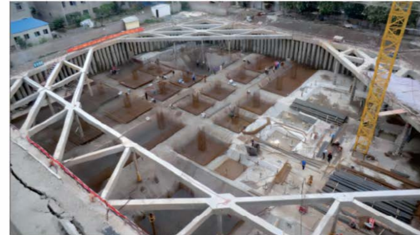
Deep foundation pit
