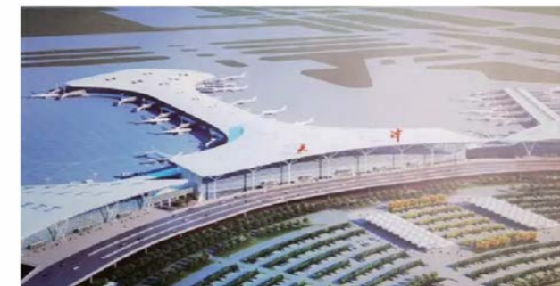
Tianjin Binhai International Airport Project
